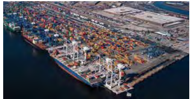
Improvements to the Howard Street Tunnel would ensure future growth at the Port of Baltimore (pictured). Photo Credit: Bill McAllen
